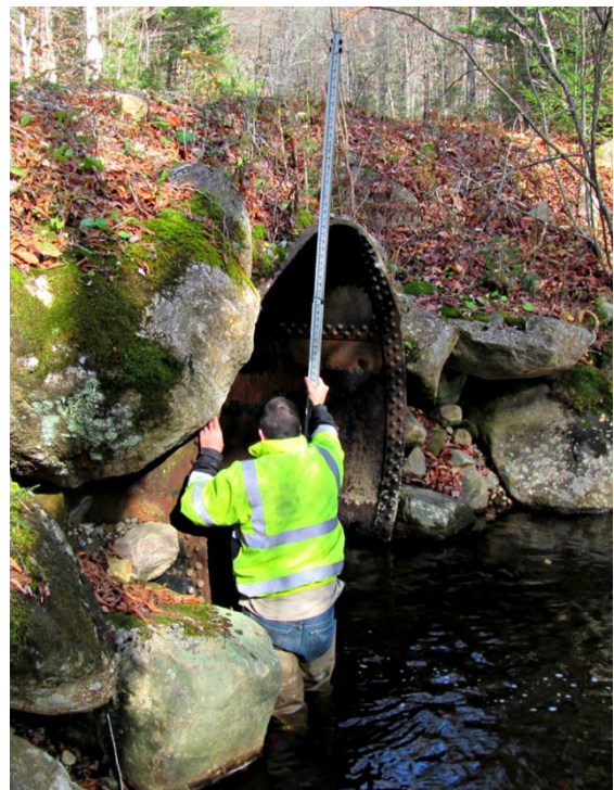
Technician Lenny Croote takes measurements during a culvert survey.
