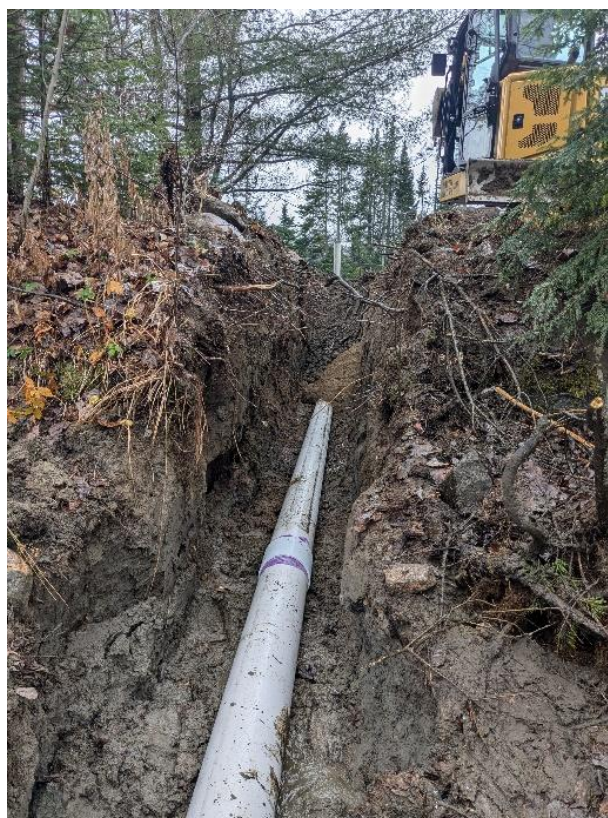
Dry hydrant repair project
