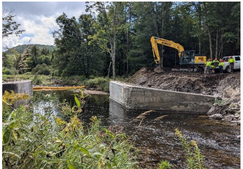
Robb’s Creek Bridge Repair Project, Town of Wells
