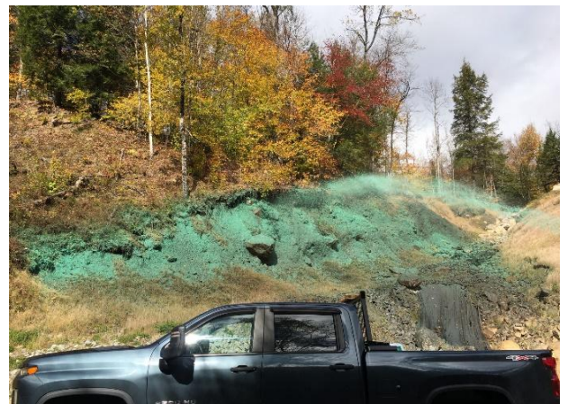
Hydroseeding the steep banks of Gilmantown Road, Town of Wells
