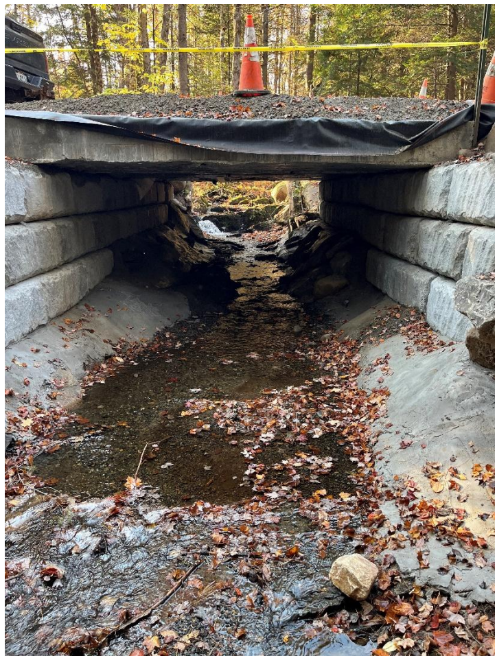
Bear Creek Culvert Replacement Project, Town of Hope
