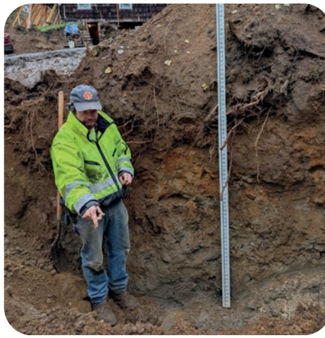
← Sr. Technician Lenny Croote conducts a perc test for a landowner installing a septic system.
